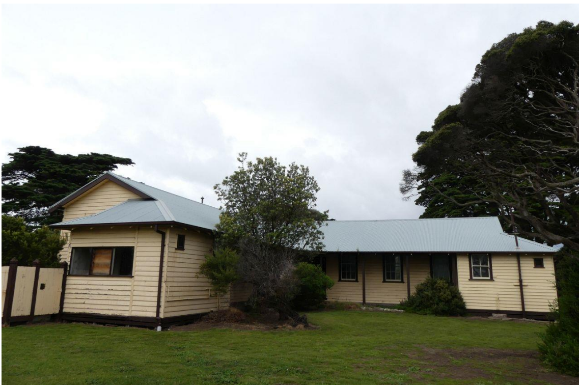
Figure 7 Building 66, the former isolation wards, viewed from the north-west
